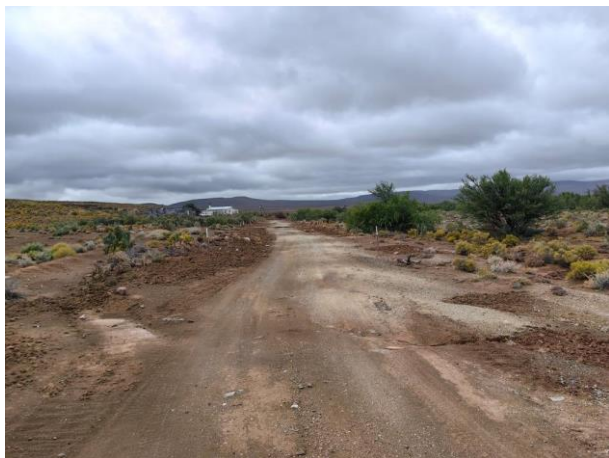
Road construction underway.
